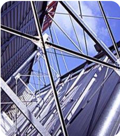
Figure 1: Structure Contreventée
